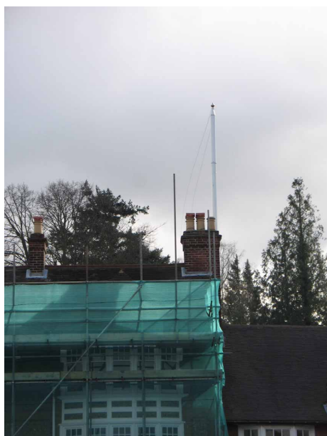
Picture 6.6 This mast in Sunningdale is designed to look like a flagpole.
