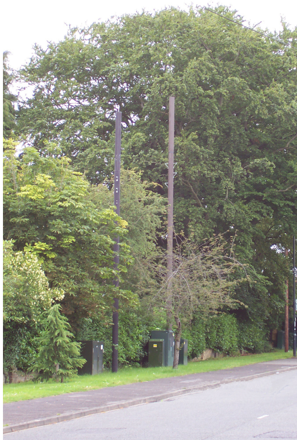
Picture 6.2 The visual impact of these masts has been minimised by their siting with a backdrop of trees and their design to appear like telegraph poles
