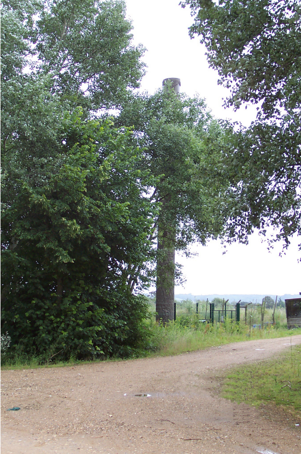
Picture 6.4 This mast near Cookham has been disguised to appear like a tree trunk
