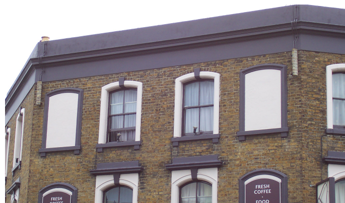
Picture 6.7 These cells on a building in Maidenhead have been designed to blend into the appearance of the building.
